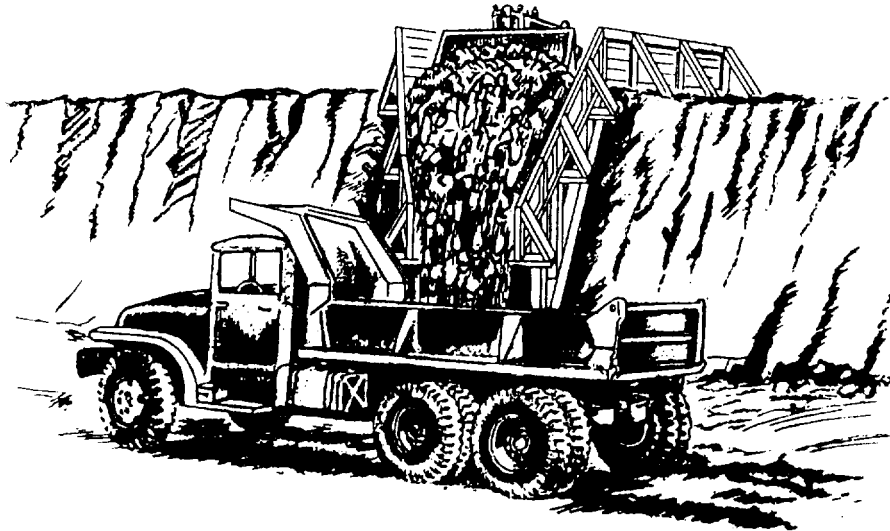
Figure 5-7. Plain chute loading ramp.
